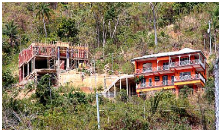
New houses being built on the mountains. Photos: Jennifer Watson
